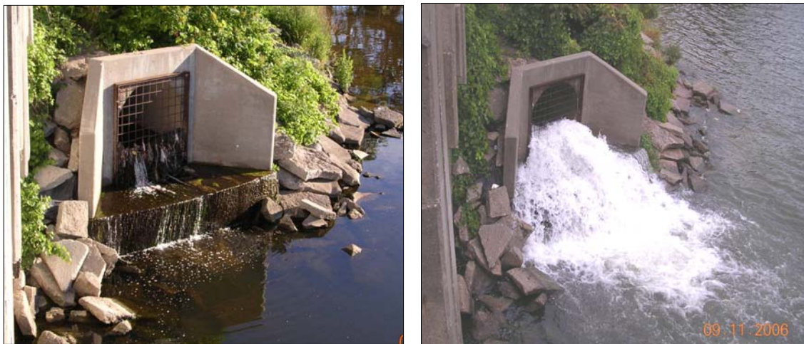
Figure 1. Stormwater discharge from a storm drain entering Mona Lake (Norton Shores, MI). Drain on left is under dry conditions, whereas drain on right is after a 1-inch rain event. Photo credits: Alan Steinman (left); Annoesjka Steinman (right).
